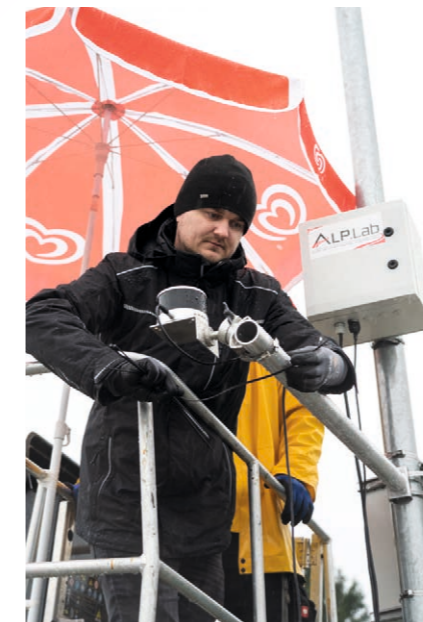
Image 8: Wiring the lidar sensor ©AustriaTech/Schallauer
